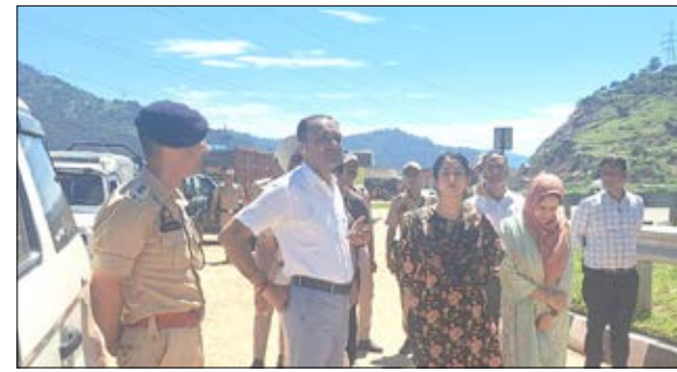
of the Jammu-Srinagar National Highway NH-44 at Thard to take stock of the ongoing restoration works.
